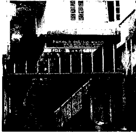
Santhivilla Pump House
