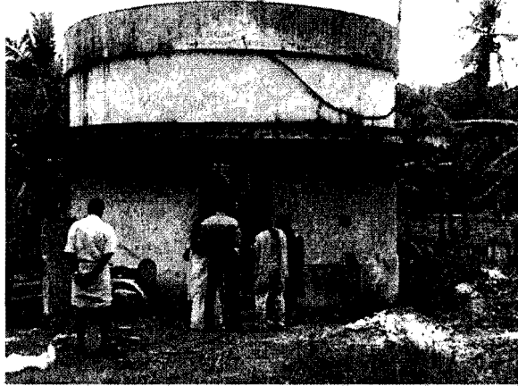
Kakkamoola Pump House
