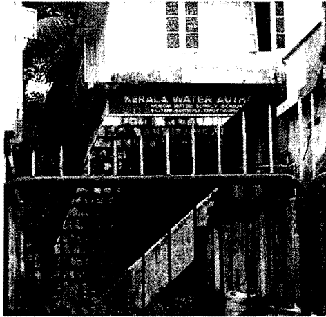
Santhivilla Pump House
