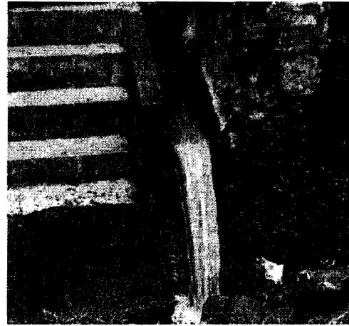
Over Flow of Water from the Pump House
